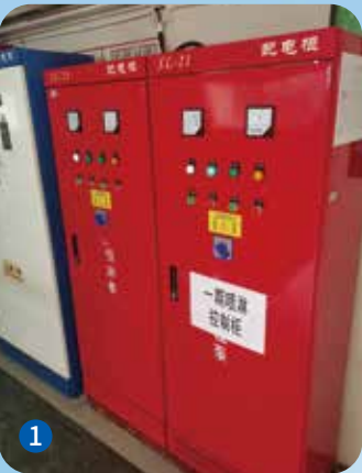
1 Firefighting sprinkler control cabinet
